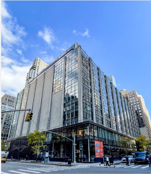
Wide Curtain Wall
