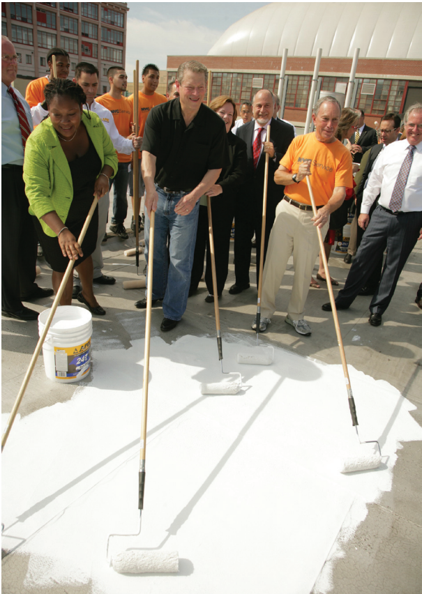
EF 11: White roofs are an inexpensive way to reflect heat away from our cities.
