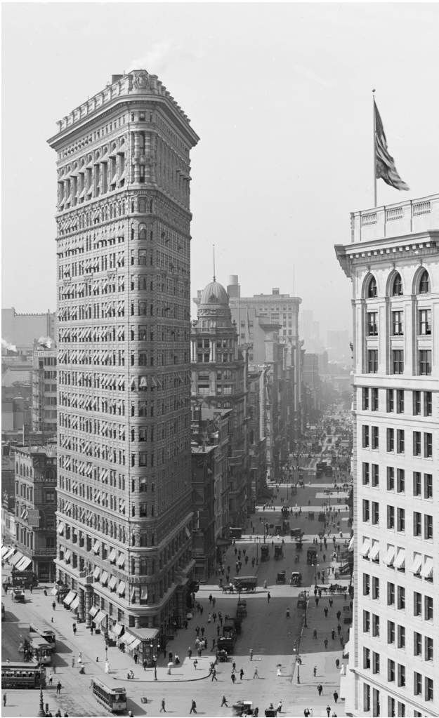
EF 6: Solar shades were a common feature in New York City prior to the advent of air conditioning systems, as seen in this photo of an awning-encrusted Flatiron building.
