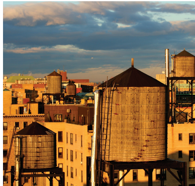
BR 8: Rooftop water towers have long been a fixture of the New York City skyline and, unlike pump driven systems, can help ensure access to potable water during a crisis.
